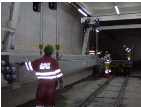
Bankettelement (11 t schweres 10 m Element)
