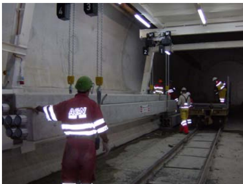
Bankettelement (11 t schweres 10 m Element)
