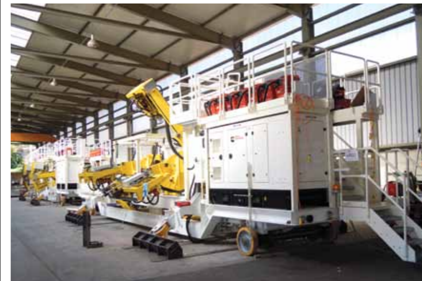
Above: Two Rowa rigs were used to drill the array of more than 250,000 holes required for services on the project
