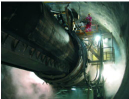
Shotcrete robot in the area LZ
