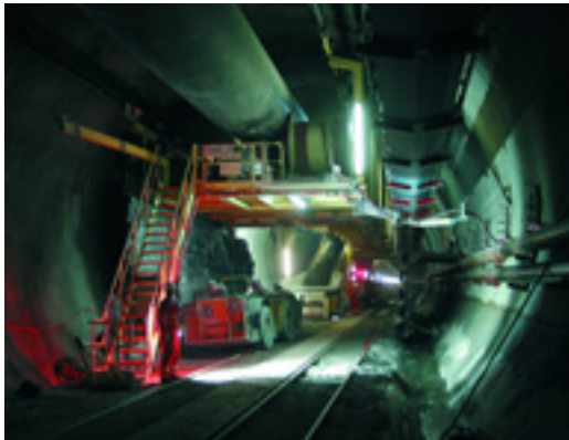
Cross passage installation
