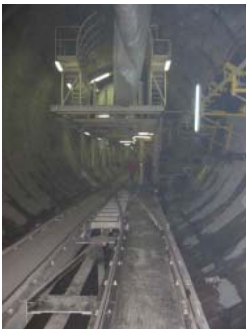
Rear of the back-up system with front of the rolling platform
