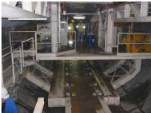
Lining segment magazine with material transloading area
