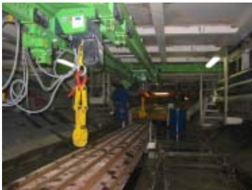
Rail-laying area with stockage of the daily requirements
