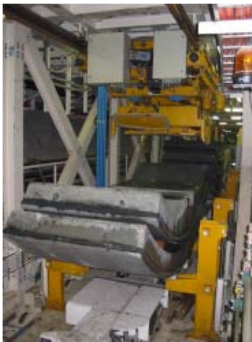
Segment unloading, lining segment transloading crane with vacuum gripper
