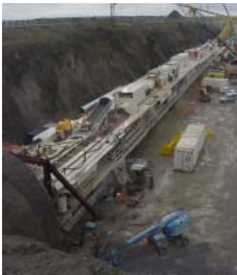
Assembly at the construction site at the northern tunnel entry, autumn 2002
