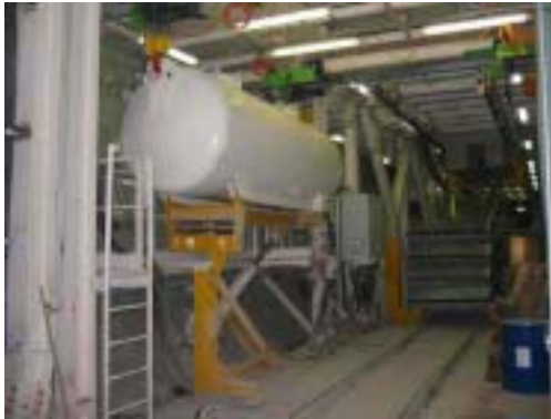
Dry mortar transloading and intermediate storage for bottom segment back-filling
