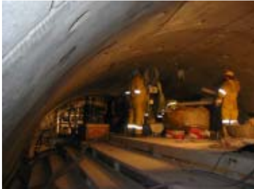
Workplace for the back-filling of lining segments
