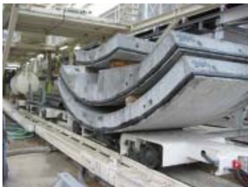
Pile of segment linings on the supply train
