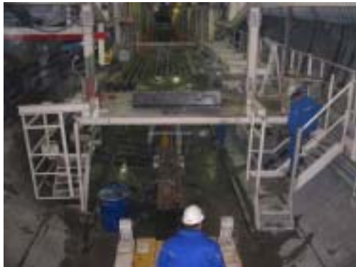
Stockage and installation area of pipes
