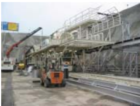
The installation is leaving day-light
