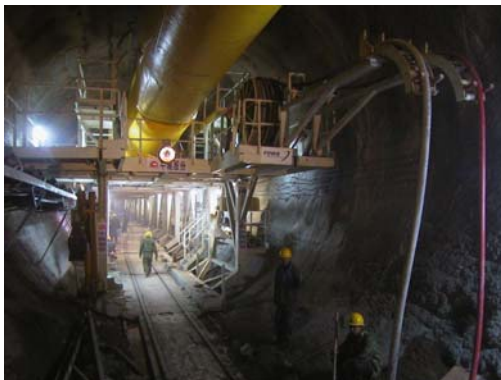
Ventilation reservoir / high-voltage drum
