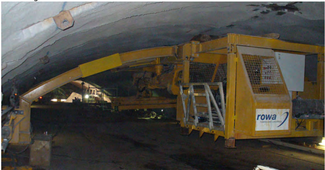
Picture: Overhead traveling crane
