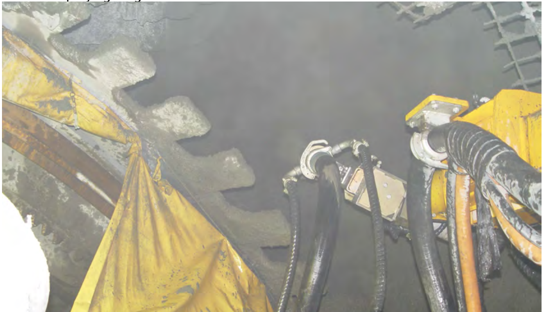
Picture: Shotcrete robot L1 immediately behind flight conveyer
