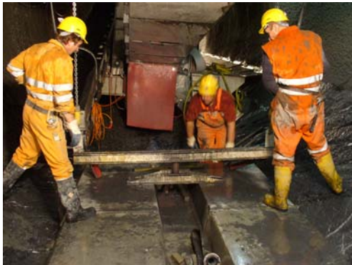
Base segment-installation with lining segment transloading crane
