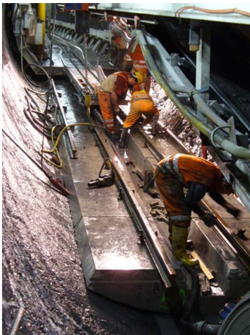
Track installation bridge at the front tongue
