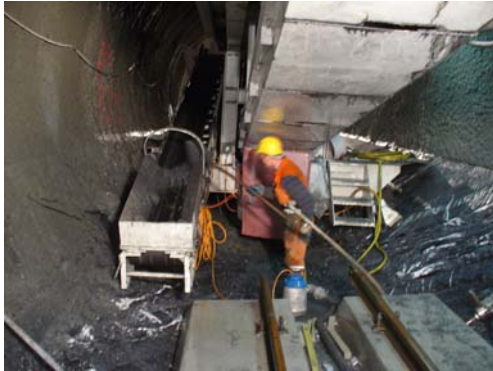
Invert cleaning conveyor
