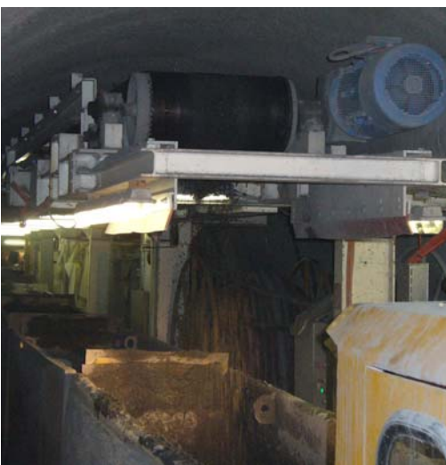
Transfer back-up conveyor into muck car
