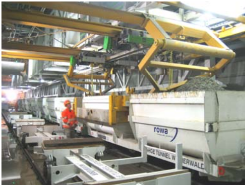
Unloading of invert concrete transport container (4.5 m 3 ) with special crane.
