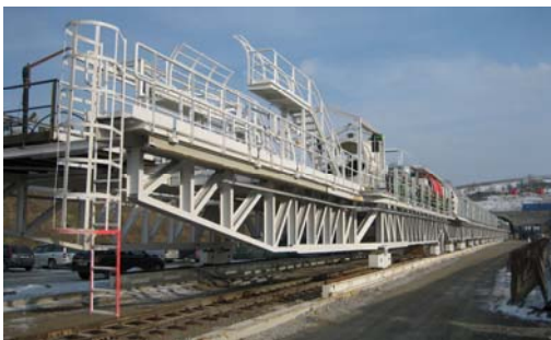
Back-up installations ready for the heading
