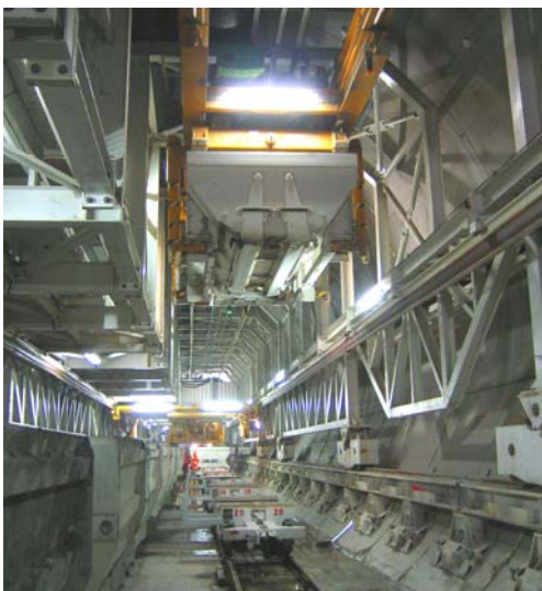
Simultaneous transloading of sand and bonding agents with invert concrete transloading.
